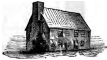
Whitefield’s House, as seen from the west.
